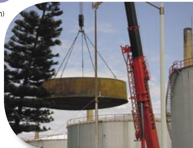
*The new bottom for tank 1805 is lifted into place.*
