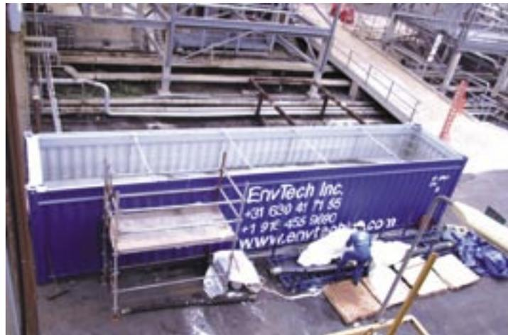
During the recent shutdown of the alkylation unit, it was chemically cleaned using the EnvTech process which clears all iron fluoride scales accumulated in the unit. Here, we see the container that was used to mix the buffer solution.
