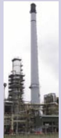
Work has started on the maintenance and painting of SAPREF's seven concrete stacks, with the first one, at north zone, complete. It is now a pleasing light grey colour.
